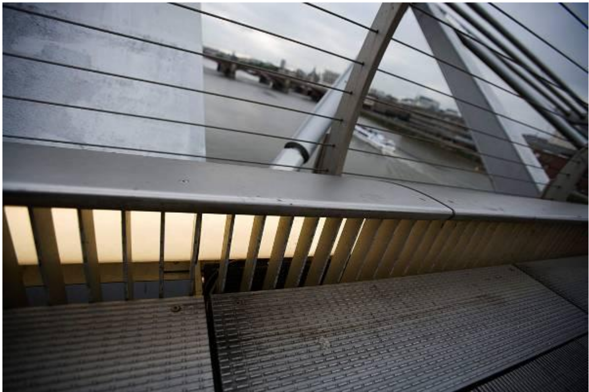
Installation point on Millennium Bridge.
